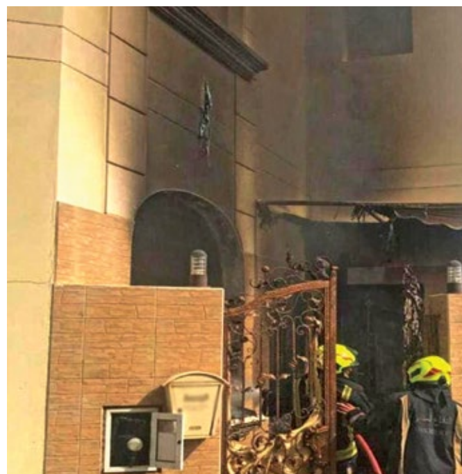
A section of the house that caught on fire
